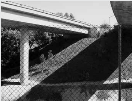
Chad Riss, Rose Creek Bike/Pedestrian Bridge, San Diego, California, 2009 .
